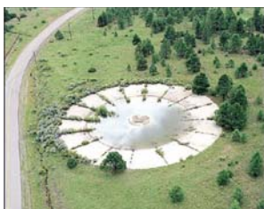
This “concrete bowl” was built at Los Alamos in 1944 and used in plutonium recovery tests.
