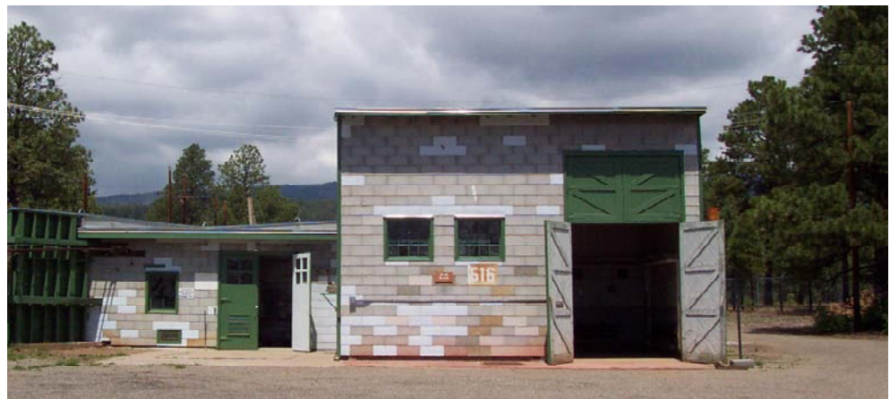
The "V-Site" High Bay Building where the Trinity device was assembled.
